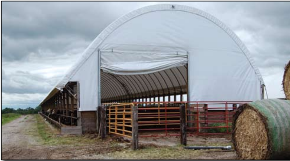
Hoop confinement building
